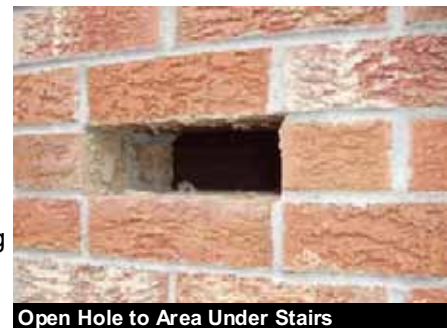
Open Hole to Area Under Stairs
