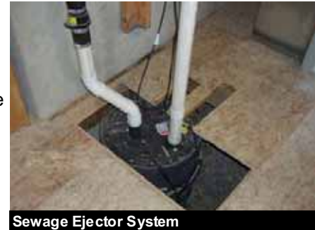
Sewage Ejector System
