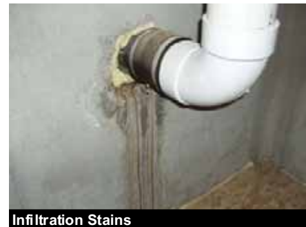
Infiltration Stains
