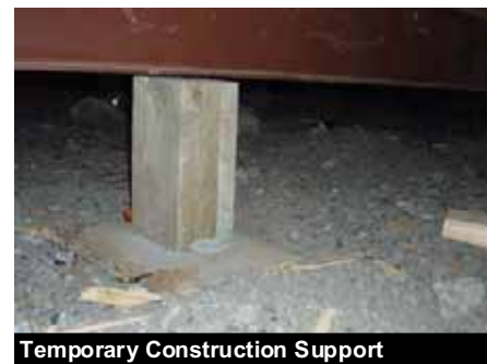
Temporary Construction Support
