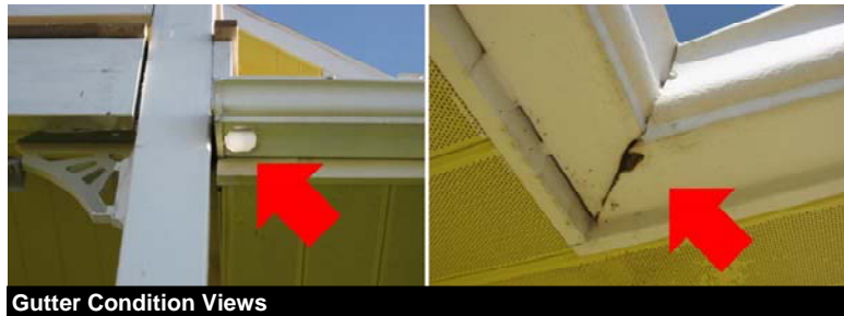
Gutter Condition Views
